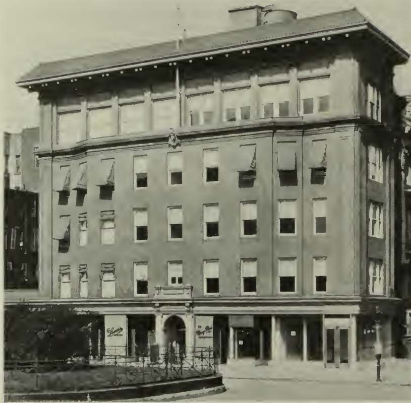
APARTMENT HOUSE, PARK AVE., NEW YORK. Built of buff Devonshire brick made by the Kittanning Brick & Fire Clay Company. Pfothenhauer-Nesbit Company, New York Representatives. Headman & Schoen, Architects.
